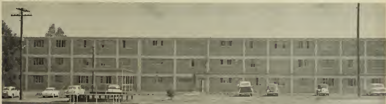
THE MODERN barracks at Naval Communications Station, Asmara are shared with Army personnel stationed there.
